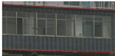
The second floor long window
